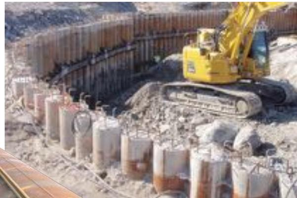
Installation using flexible strong WOM/WOF connections are simplified by the use of a template and panel installation method.
