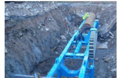
Example of tunnel using O-Pile®:DTH using horizontal drilling. While vertical walls are assembled with standard DTH piling rigs, horizontal applications require special HZ rigs that can handle long element lengths as the space allows.
