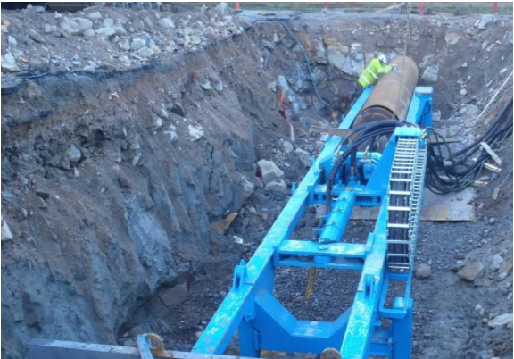
Example of tunnel using O-Pile®:DTH using horizontal drilling. While vertical walls are assembled with standard DTH piling rigs, horizontal applications require special HZ rigs that can handle long element lengths as the space allows.
