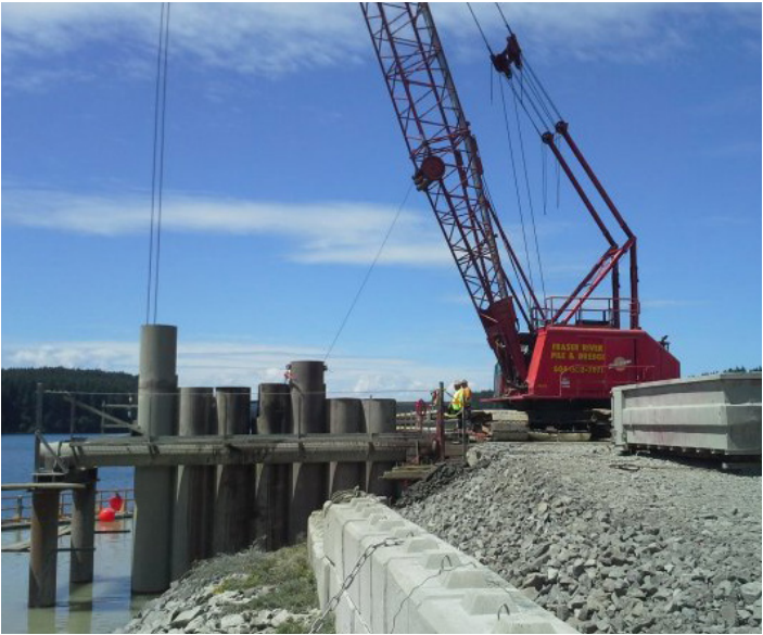
O-Pile® template in marine environment.
