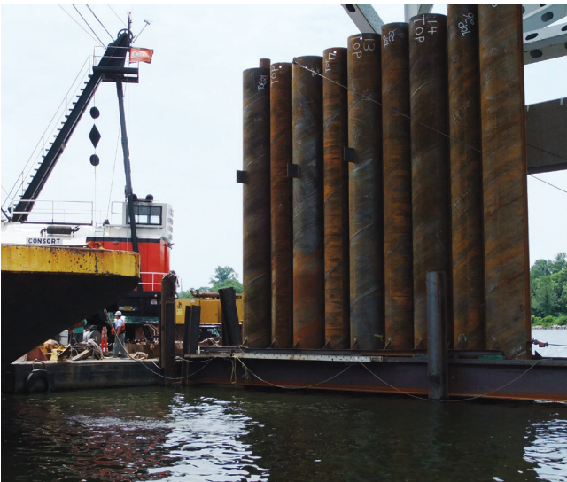
Picture illustrates the superior template and panel installation method that O-Pile systems utilize.
