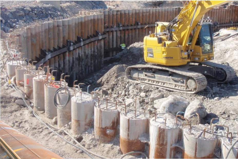
FIGURE 4 DTH-O-Pile The Only SSP System that Can Be Driven Through Solid Rock.
