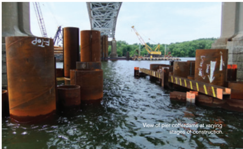
This panel was assembled and moved into position under the bridge due to limited headroom.
