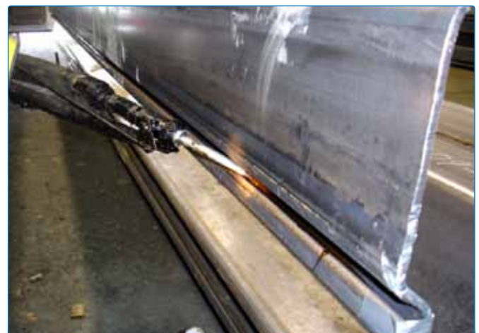
Figure 2. Wadit can be quickly and efficiently applied into any steel sheet piling interlock including cold formed sheets like that above.
