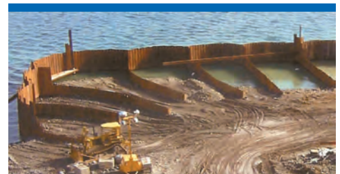
A USCG open cell dock with 70 foot face sheets under construction in Unalaska, AK.
