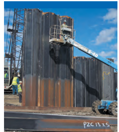
IHNC Levee Rebuilding, New Orleans
